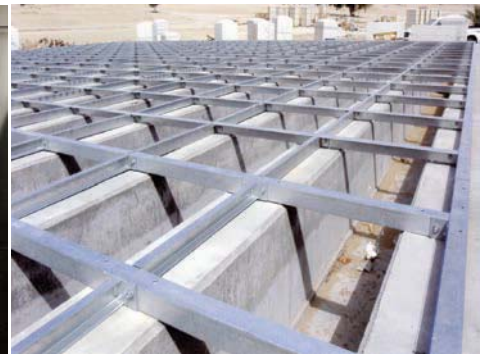
Base Frame Foundation
