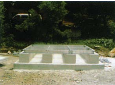
● Concrete Base & Foundation
